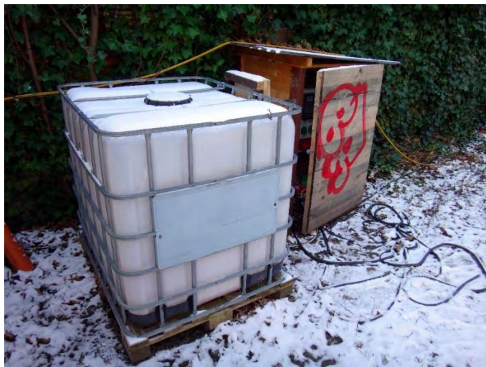
Figure 16 - BD's improvised electric box (source: author)
