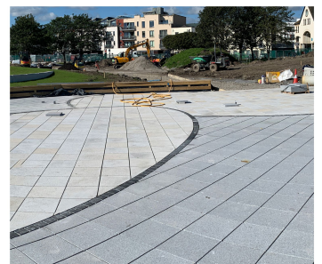
Estuary Area under construction
