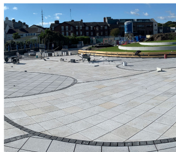
Estuary Area under construction
