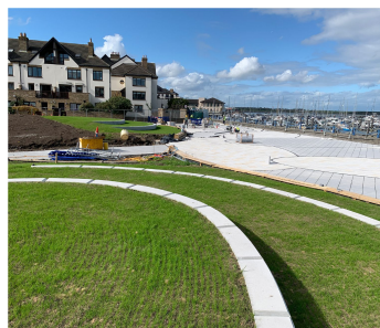
Grass terraces - Under construction
