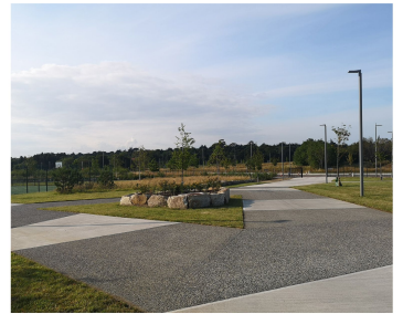
Paving Detail - Variety of concrete finishes
